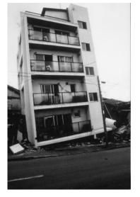
Medium rise reinforced concrete shear wall buildings without moment resisting frames (#8) Reinforced concrete shear wall without moment resisting frame, high rise (#9)
